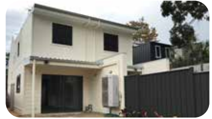
ABORIGINAL HOUSING OFFICE $1.2m Waterloo, NSW
